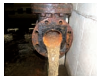
This picture was taken during a building water meter replacement
